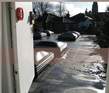
*This door marked as fire exit, lead directly onto a flat roof with no means of getting to the ground level beyond jumping!*
