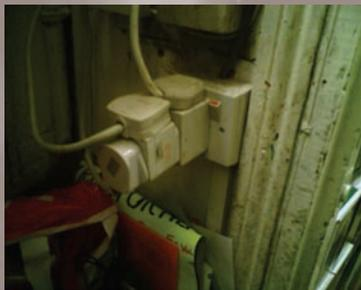
*These electrical 'cube' adapters were 'piggybacked' into each other resulting in a heavily overloaded socket, a highly unsafe practice.*
