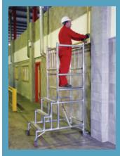
seems to show that the misuse of low level access equipment is commonplace with users frequently climbing up the wrong side, not using locks to make the structure rigid, not using safety gates, not using the brakes on the wheels of the platform and using mid-level
