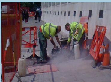
*These workers were seen using a skilsaw on the pavement with no eye protection, dust mask or ear defenders.*
